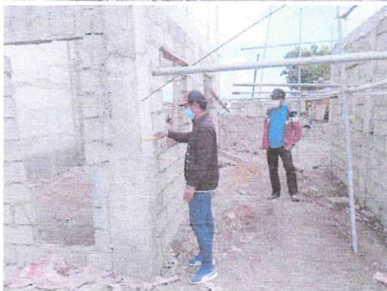
Site Visit & Inspection of the team
